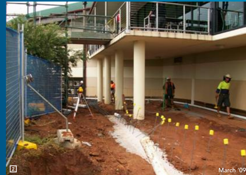
2: Golf Club Refurbishment
